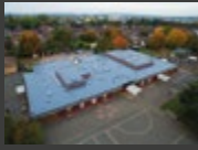
LIQUID APPLIED ROOFING
